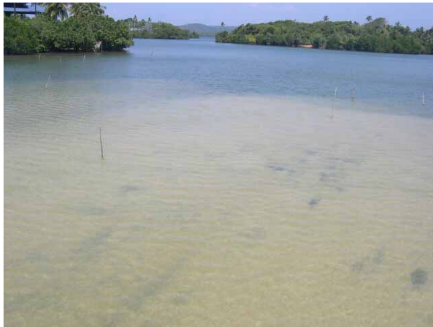
Kogalla Lagoon. Siltation under the Kattalue railway bridge.
