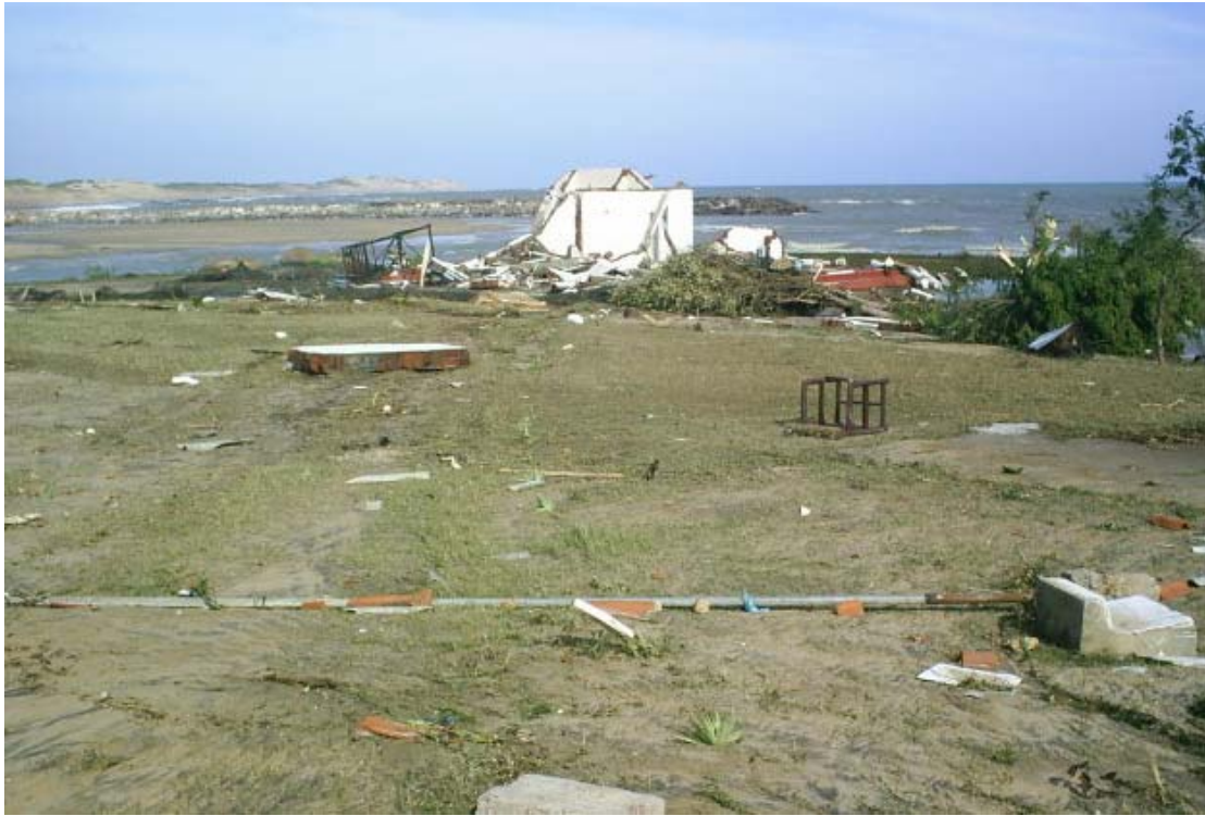
A damaged house in Hambantota District Source: GMSL
